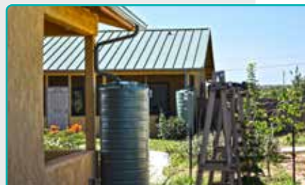
WATER STORAGE TANKS
